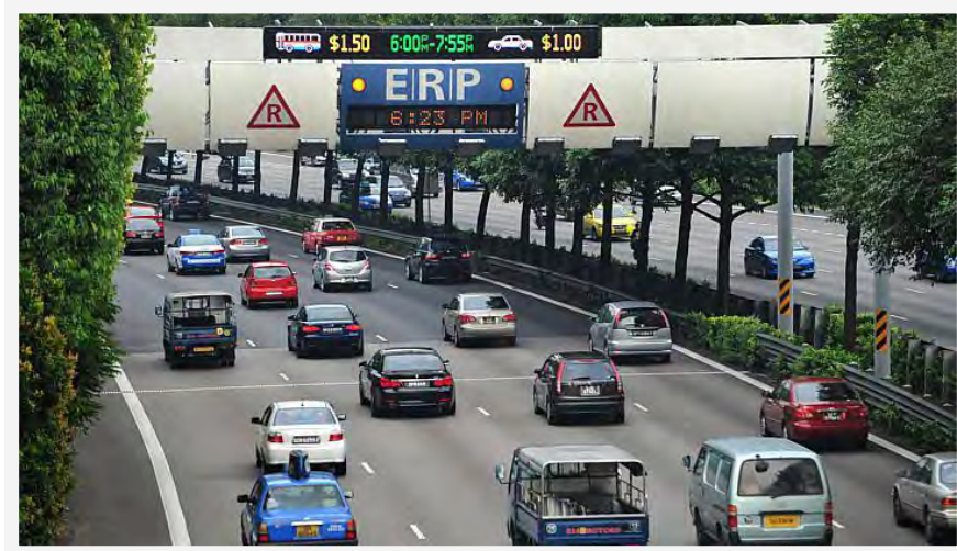
Figure 7. Toll collection in Singapore using Automatic Number Plate Recognition (ANPR)
