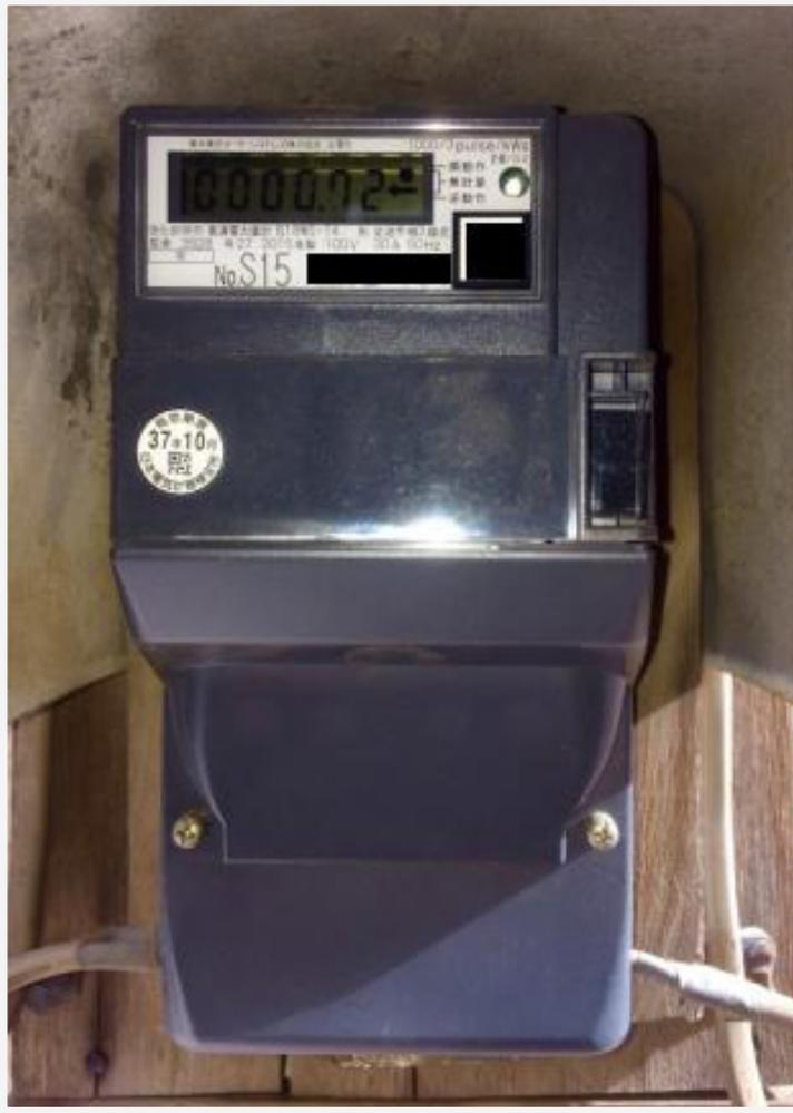
Figure 4. Smart meter that supports Route B services in Tokyo
