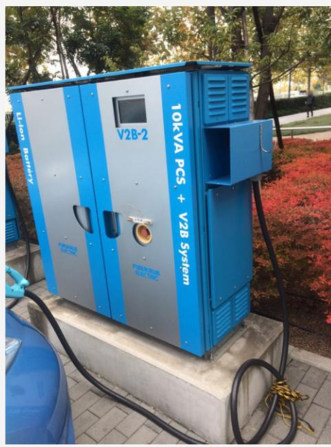
Figure 8. Vehicle-to-building (V2B) system used in Yokohama
